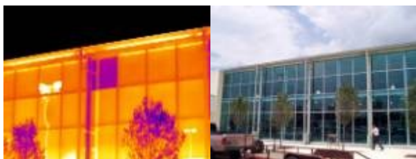
Thermal image of double pane window versus single pane windows – clearly showing the difference in energy efficiency.
